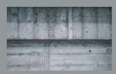
Original 1960s concrete ceiling with the formwork (wood grains) still visible. With part of the building's history. This can also
